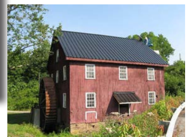
The new roof being completed on the Mill in 2008.
